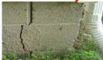
CRACKED FOUNDATION
